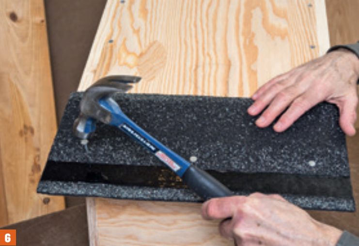
6. Install each starter shingle so it overhangs the decking by about ¼" and the adhesive strip is near the bottom (eave) edge of the roof. 7. Nail the shingles just above the level of the tab slots so the nails are covered by the next row of shingle.
