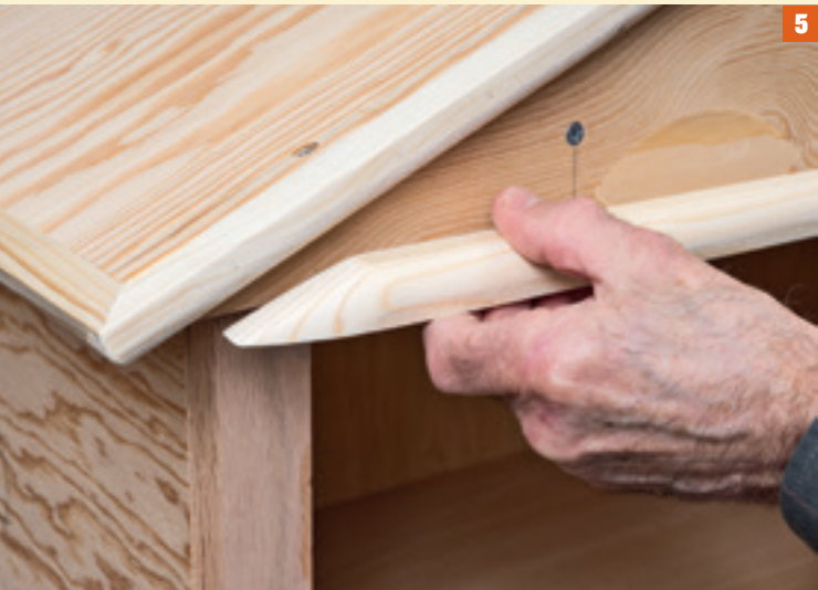
4. Position all roof deck trim so the rounded side of the molding faces out. 5. Cut the horizontal trim to fit the gable slope, then bevel the cut for a finished look.
